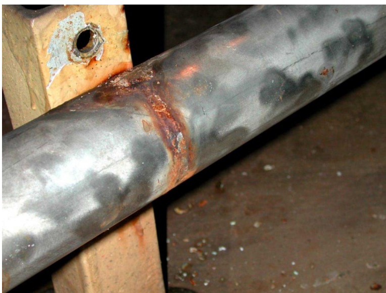
PHOTOGRAPH 2 Pits Forming as a Result of Crevice Corrosion between the U Bolt Support and the Pipe
