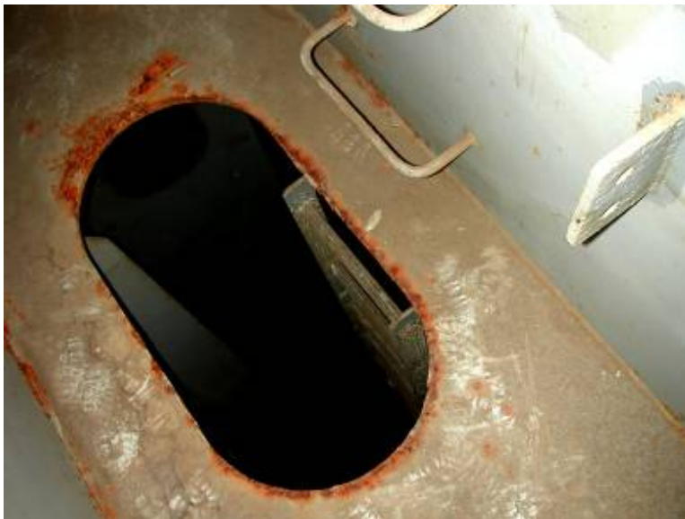
PHOTOGRAPH 17 Coating Breakdown around Cut Out
