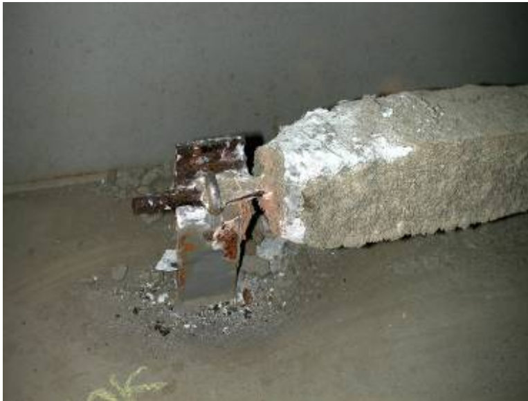
PHOTOGRAPH 1 Normally Working Anode
