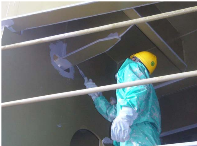
PHOTOGRAPH 18 Stripe Coating Application (1 January 2017)
