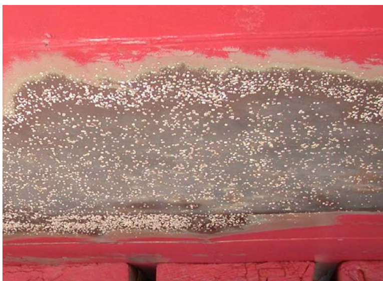
PHOTOGRAPH 2 Early Stages of Barnacle Fouling on an Area Where the Anti-fouling Paint had been Damaged
