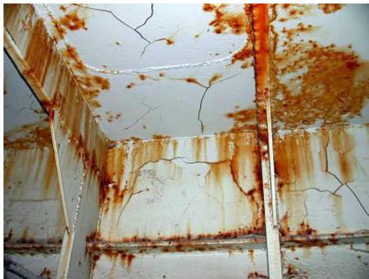
PHOTOGRAPH 25 Typical Mud Cracking in a Thick Coating
