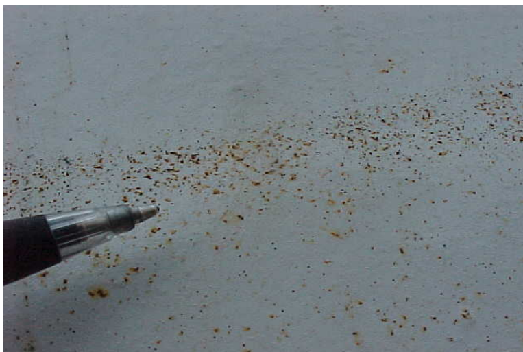
Trapped Grit at the welds and in the coating has caused rust staining. Grit that penetrates through the coating allows corrosion of the substrate to initiate.
