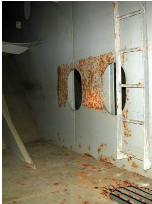
PHOTOGRAPH 15 Example of Poor Surface Preparation Prior to Coating
