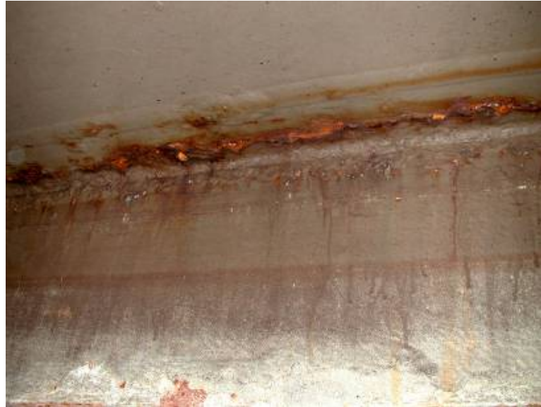
PHOTOGRAPH 18 Corrosion around Weld
