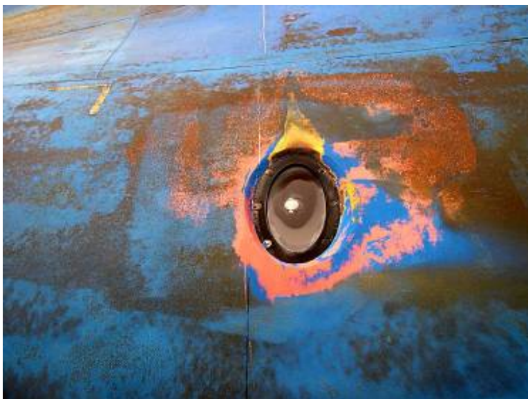
PHOTOGRAPH 7 An Example of an ICCP Anode on a Ship
