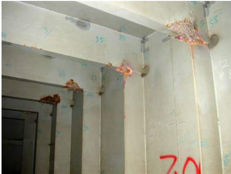
PHOTOGRAPH 26 Stress-induced Coating Failures
