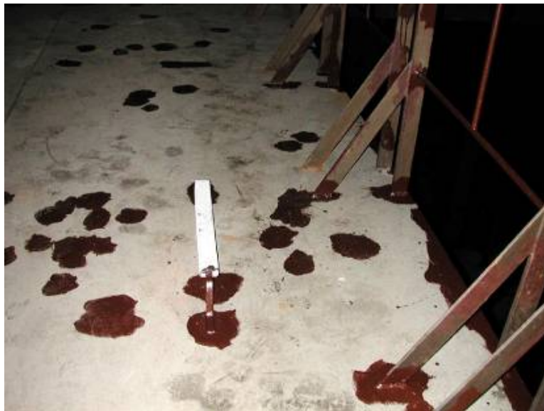
PHOTOGRAPH 1 Brush Applied Touch-up Paint on a Forepeak Stringer
