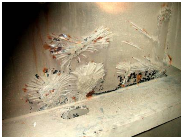
PHOTOGRAPH 22 Reverse Impact from Grab Causing Brittle Coating to Shatter
