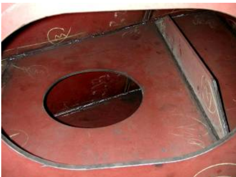
PHOTOGRAPH 11 Complex Structure, with Lower Welds Only Accessible Through the Hole
