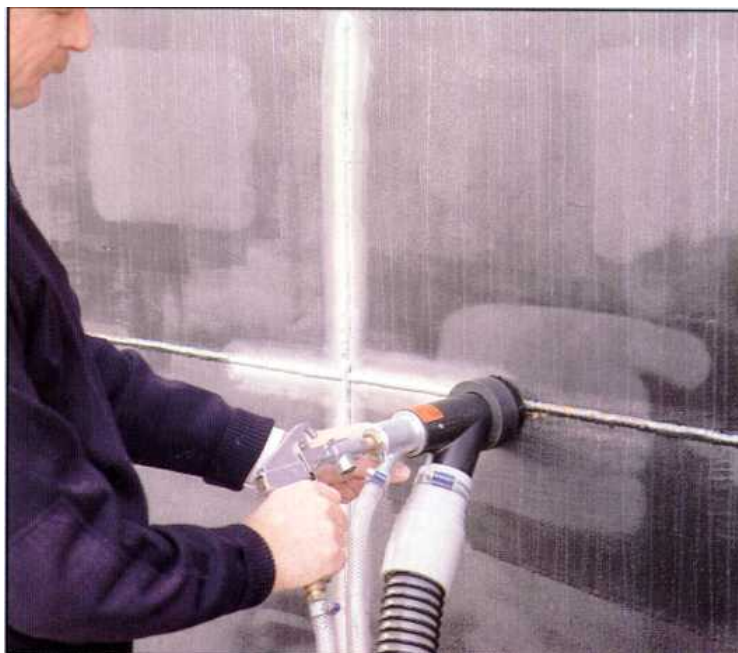
PHOTOGRAPH 16 Vacuum Blasting (1 January 2017)
