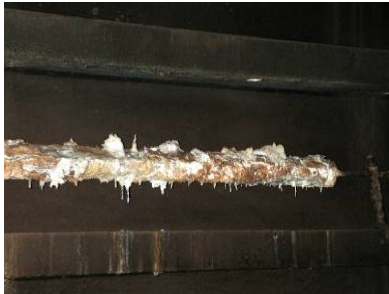
PHOTOGRAPH 3 Overworked Aluminum Anode
