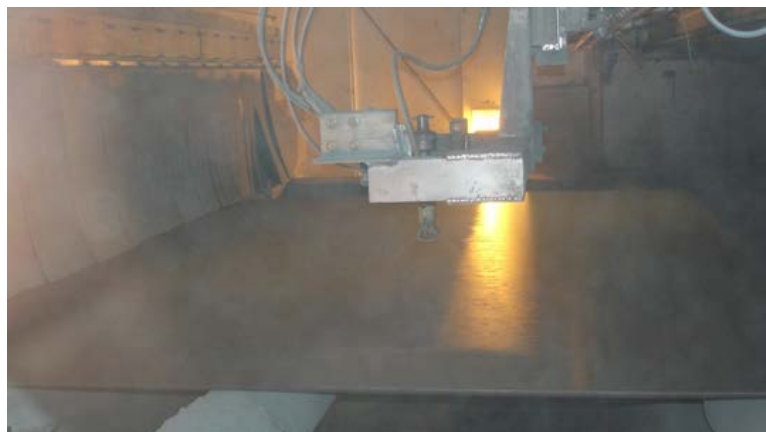
PHOTOGRAPH 11 Shop Primer Application (1 January 2017)
