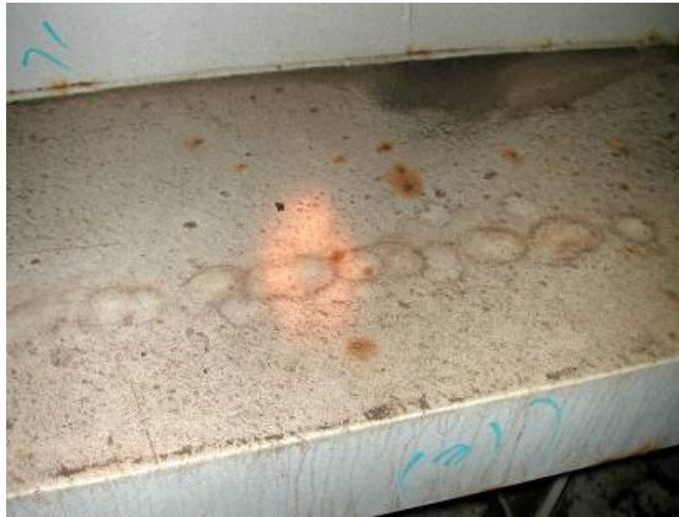
PHOTOGRAPH 11 Corrosion Spots on Longitudinal Stiffener
