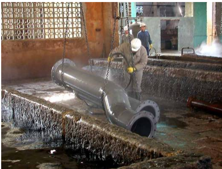
PHOTOGRAPH 8 Pipes Undergoing Pickling
