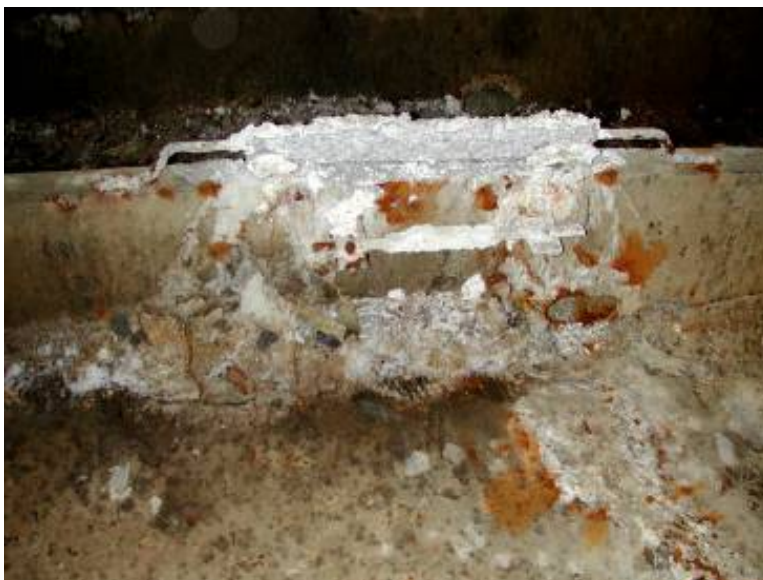
PHOTOGRAPH 2 Overworked Zinc Anode
