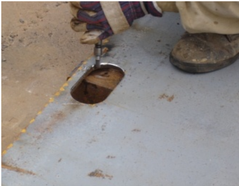
PHOTOGRAPH 14 Edge Preparation (1 January 2017)
