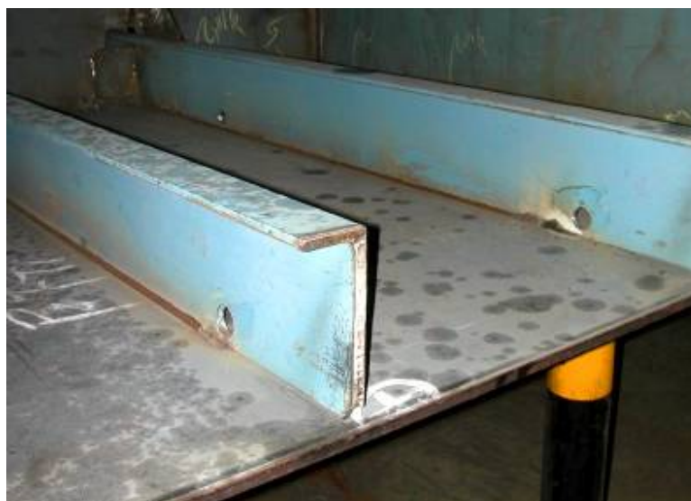
PHOTOGRAPH 3 Oil and Grease Stains during Block Assembly Show as Dark Stains on the Shop Primer
