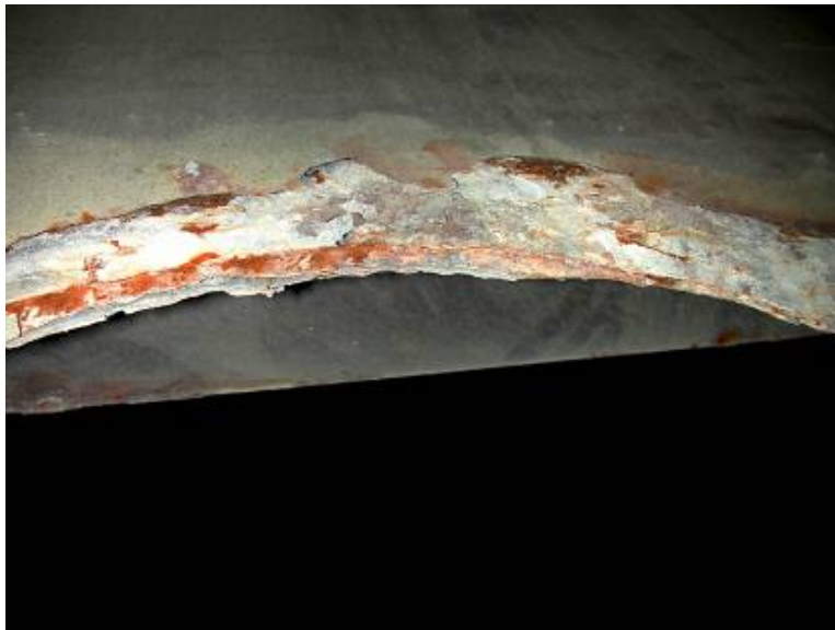
PHOTOGRAPH 20 Well-performing Cathodic Protection System with Tight Calcareous Deposits
