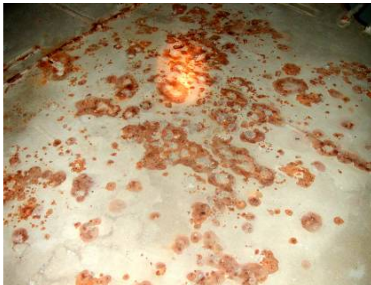
PHOTOGRAPH 12 Corrosion Spots on Stringer Deck
