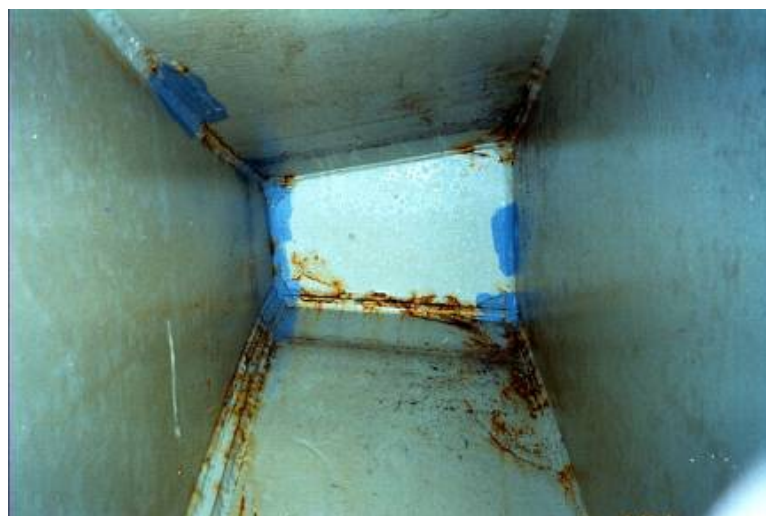
PHOTOGRAPH 19 Corrosion at Welds
