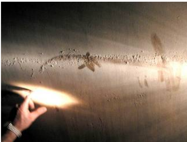
PHOTOGRAPH 10 Blistering where a Stiffener was Welded on the Other Side of the Plate
