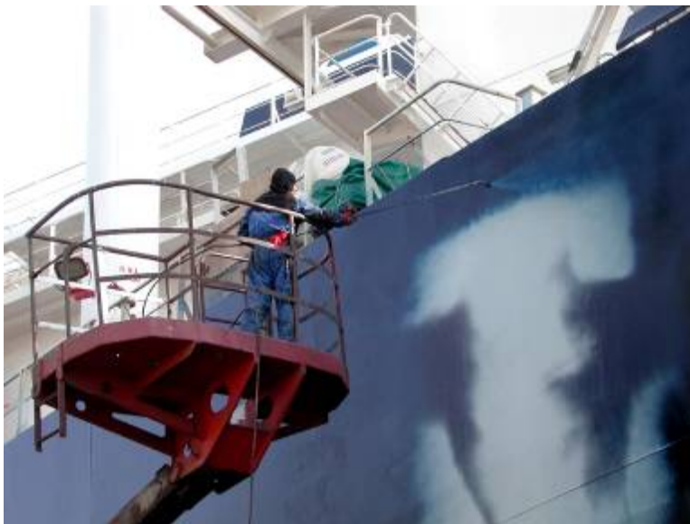
PHOTOGRAPH 3 Airless Spray Application of Paint to Vessel Topsides
