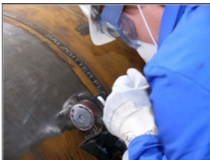
PHOTOGRAPH 15 Bristle Blasting (1 January 2017)
