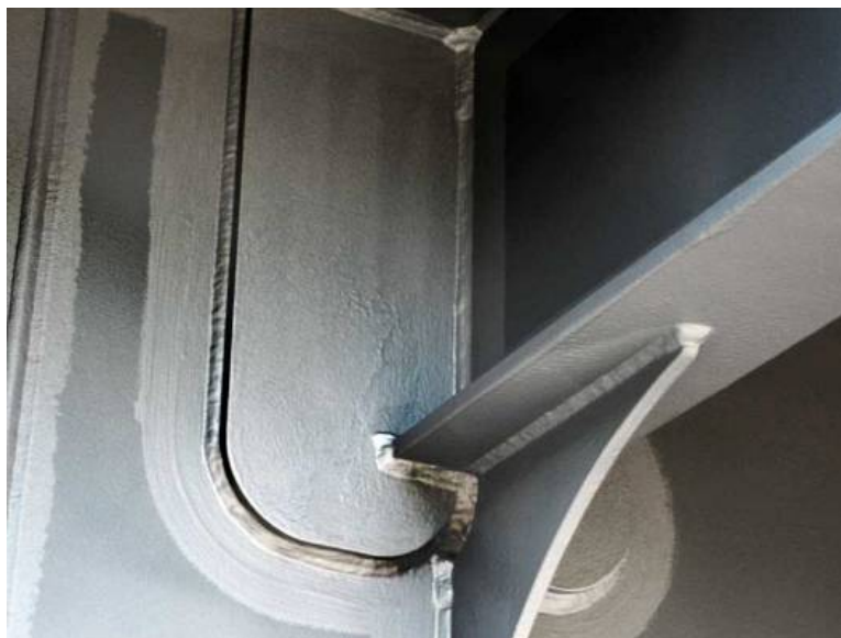
PHOTOGRAPH 2 Stripe Coating on Welded Details
