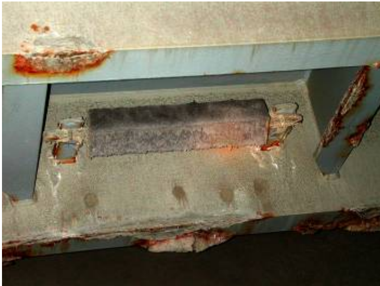
The anode is enclosed and can only protect a small area.
