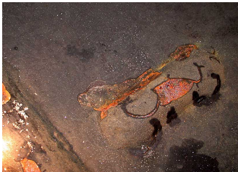
Structures in the way of tank washing systems can lose their coating and pitting corrosion can occur.
